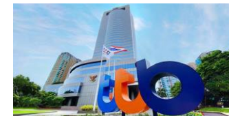
ttb bank headquarters
