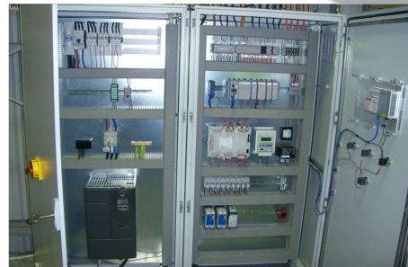
Retrofit Burner Control System
