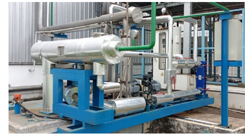
Condensate Recovery System
