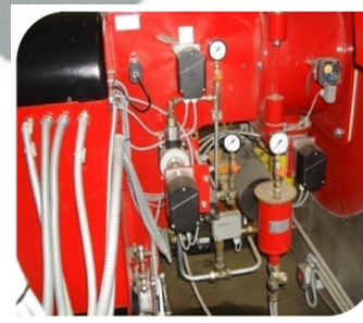
Retrofit Burner Control System
