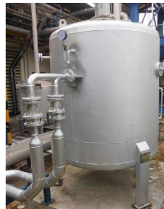
Blowdown Heat Recovery System
