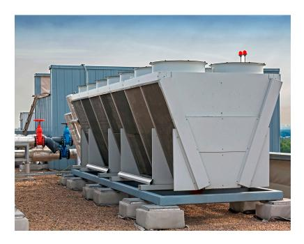
Some V-shape dry coolers have a separate adiabatic system where a water-evaporating system is added to the sides. The adiabatic system has a relatively small flow of water, either sprayed over the coil or in a panel with a fill material that provides a larger surface for the water to evaporate from. Grundfos LCSEs, VLSEs, MAGNAs and UPs could be used here. The MAGNA 3, for example, can start/stop control when the temperature is low enough not to use the adiabatic system.
