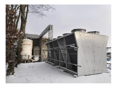
Working with a dry cooler as a cooling condenser, the general understanding is to have constant flow for the condenser and the lowest possible temperature. In cases where the dry cooler operates as a free cooler, the pump can take over temperature control in low-load situations when fan cooling isn't needed.
