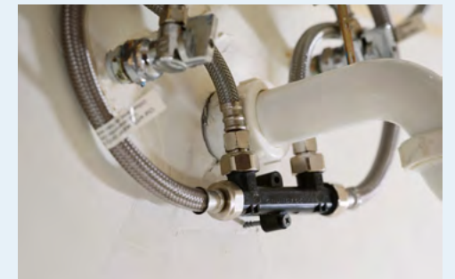
A "T" crossover valve is installed under a sink in the Stansifer's master bathroom. Along with the Grundfos ALPHA COMFORT pump, the T helps to create a loop, circulating hot water among fixtures in the home.
