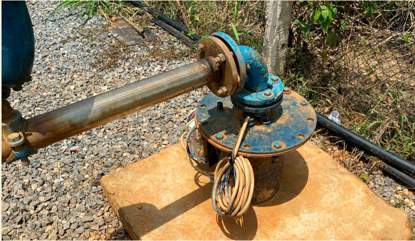
Part of the installation
