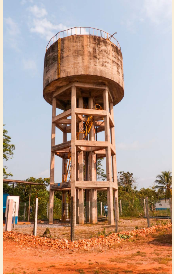
The water storage tank
