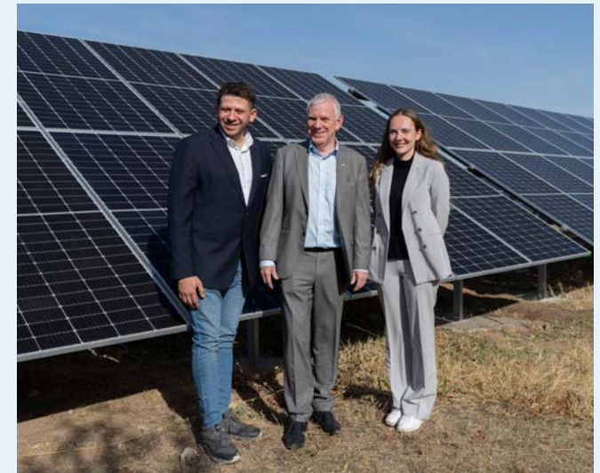
The five solar desalination systems installed around Mykolaiv desalinate an average of around 1 million litres of water every day strictly through solar power.
