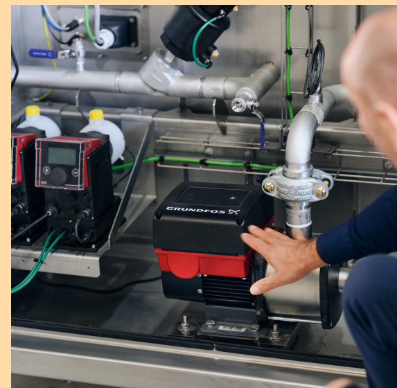
John explains the dosing pumps and the CME, which, with the integrated frequency converter, has a complete control system and can be set to pressure, temperature and flow.
