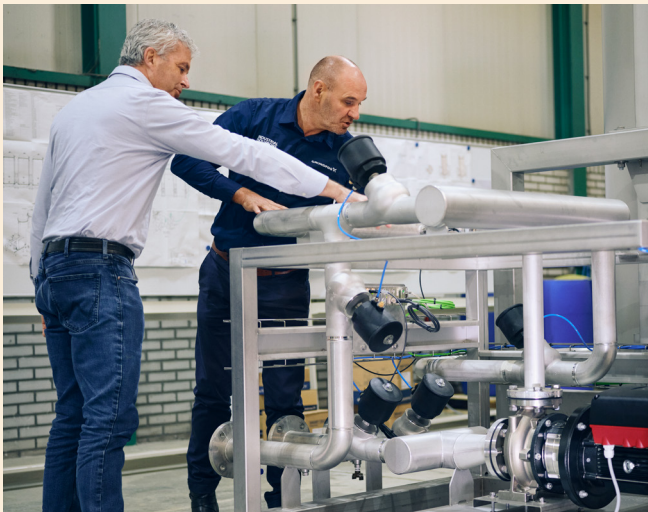
Freddy points out to John the connection of the process pump.
