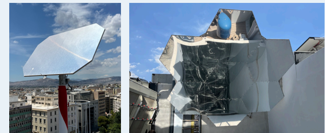
A rooftop heliostat reflects sunlight down into the building’s innovative ‘kaleidoscope’ lightwell structure.
