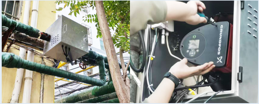
Distributed pump outdoor installation
