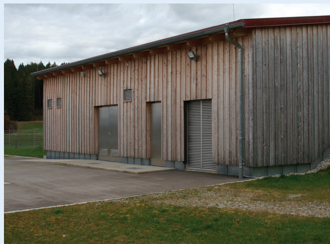
The underground reservoir comprising a technical building and two water chambers, each with a capacity of 500 m 3 , was completed in 2022
