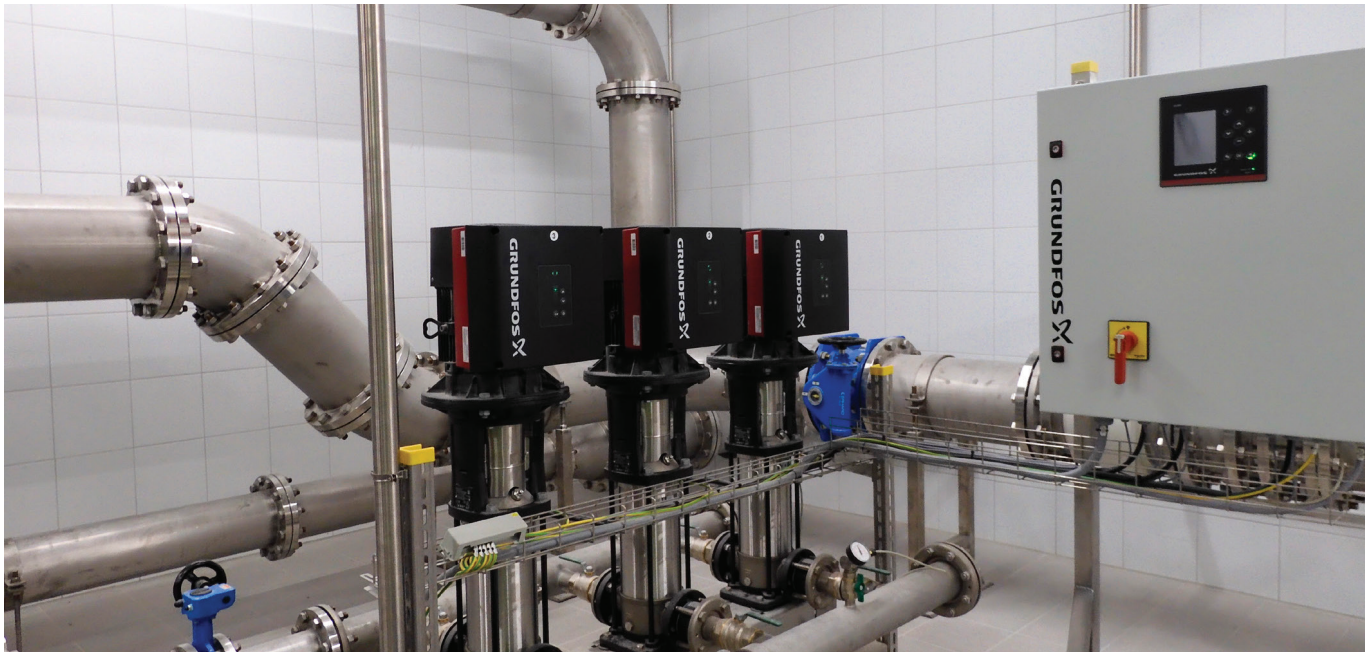
The Hydro MPC CRIE 15-7 booster system with three vertical pumps for continuous water supply
