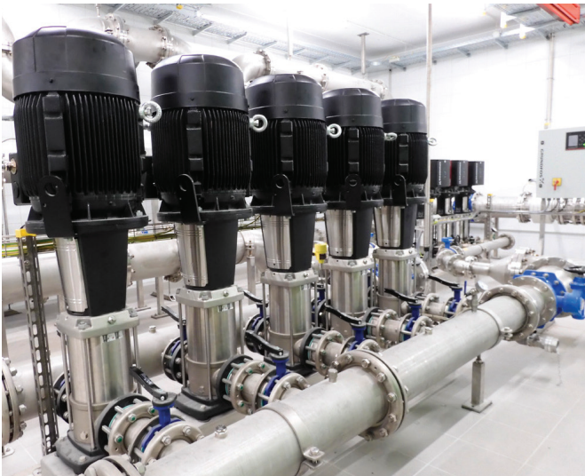
The Hydro MPC CRNE 64-3 booster system with five vertical pumps and external control
