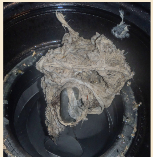
Facing clogging issues
