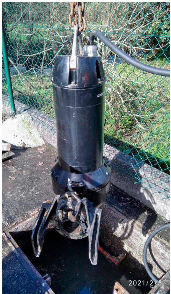
The new SL pump with Open S-tube® impeller, ready for installation
