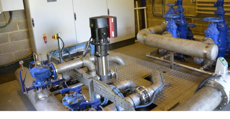
Remove existing CRIE15-09 jockey pump and replace with new CRIE 15-09 jockey pump complete with IE5 permanent magnet motor.
