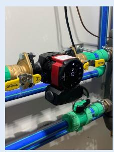
Pictured above is the ALPHA 15-58 used to push hot water through an in-floor radiant system in Kuepfer's 4,250 sq. ft. home, serving 5 zones in the house. The guided setup feature on the GO app allowed Kuepfer to easily commission the pump. The constant pressure AutoAdapt control mode is the ideal setting for a zone valve system like this one, where the pump adapts to the changing demand for heat every time a zone actuator opens or closes.
