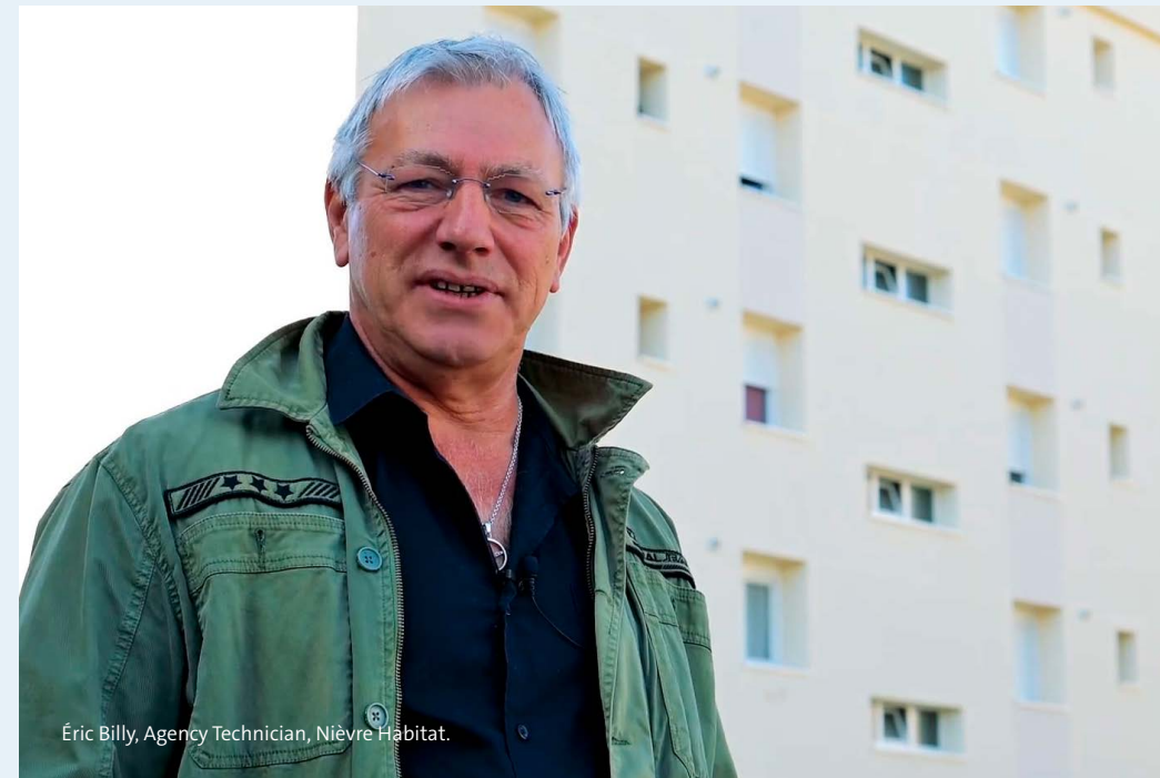
The housing complex in Cosne-sur-Loire, managed by Nièvre Habitat, which has undergone significant renovations aimed at enhancing the living conditions for its residents.
